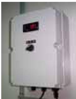
A specially designed digital temperature controller was added. It was set to cool when the temperature rose above 16° C and it turned the cooler off when the temperature dropped below 16°C.
